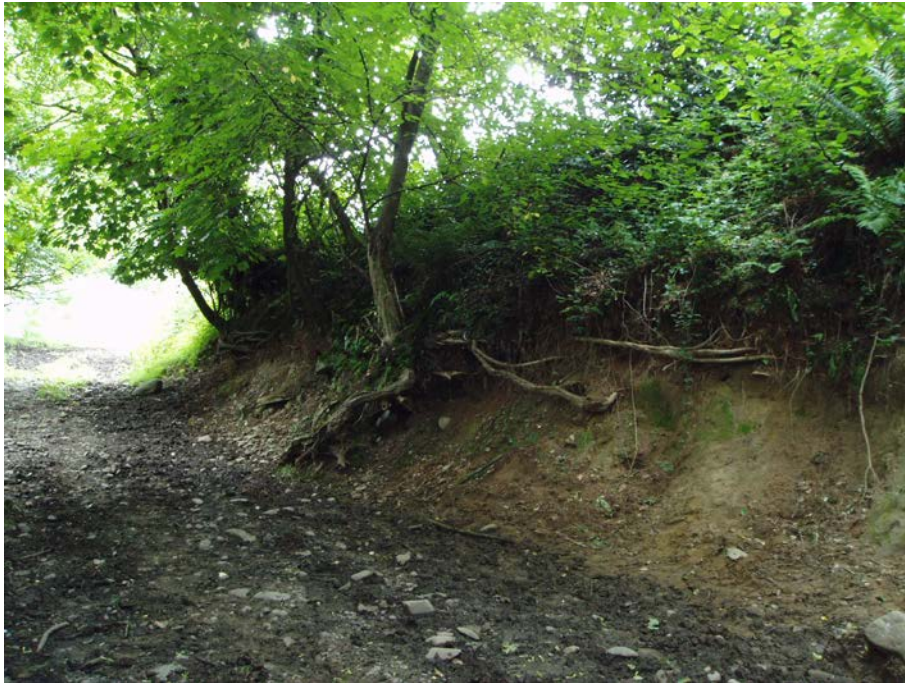
Section immediately east of the railway line on the terrace front. View looking north-east.
