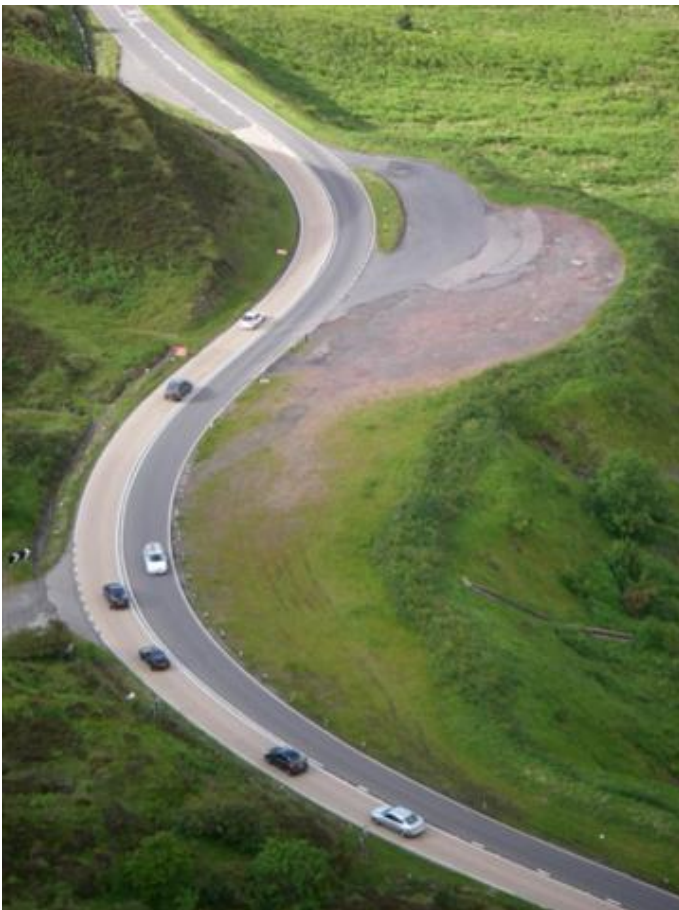
The lay-by adjacent to the Craig y Fro site – note steep slope to right dropping to the peat filled basin.
