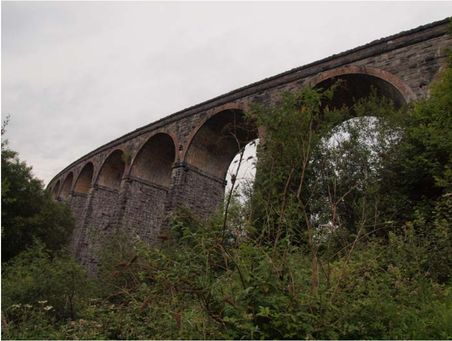
Access the site from the path below Cefn Coed Viaduct
