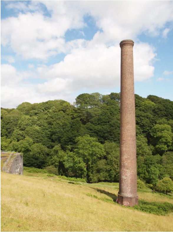
Large chimney on this site is one of the last remnants of the engine house, associated with the Henllys Vale Colliery
