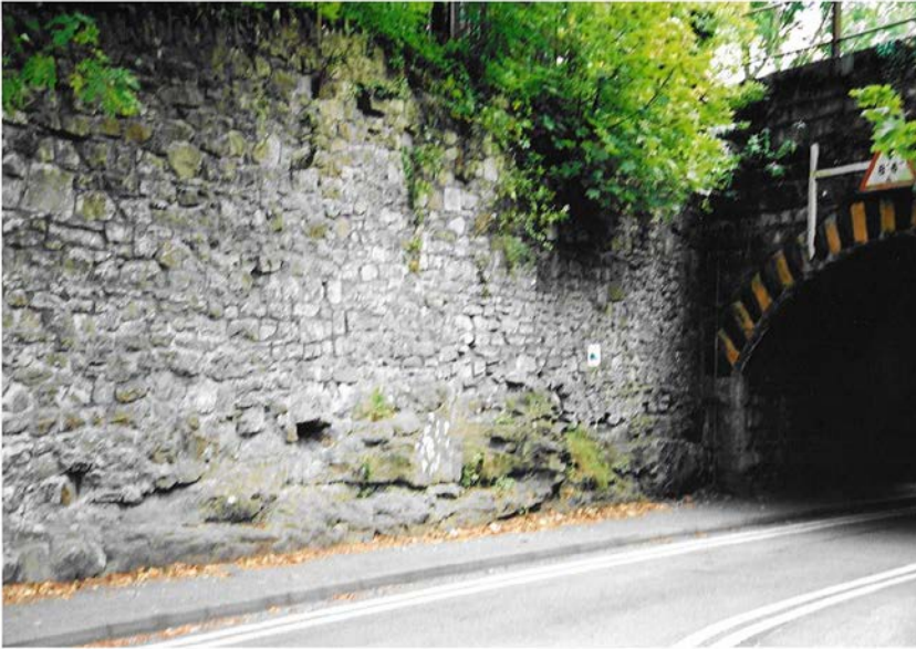
Quarella sandstone, used to build railway bridge abutments, on top of natural exposure. This example is on Quarella Road near entrance to site
