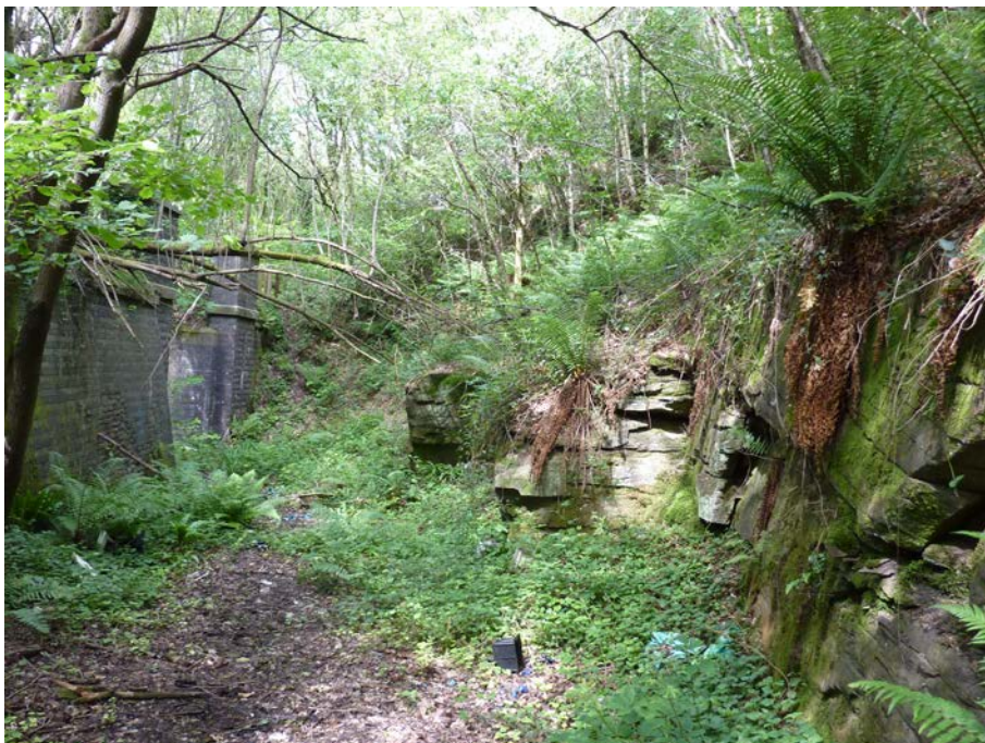
Pennant Sandstone Formation (Hughes Member) bedrock exposed at rear of terrace adjacent to former railway line View looking north at [315375 190285].
