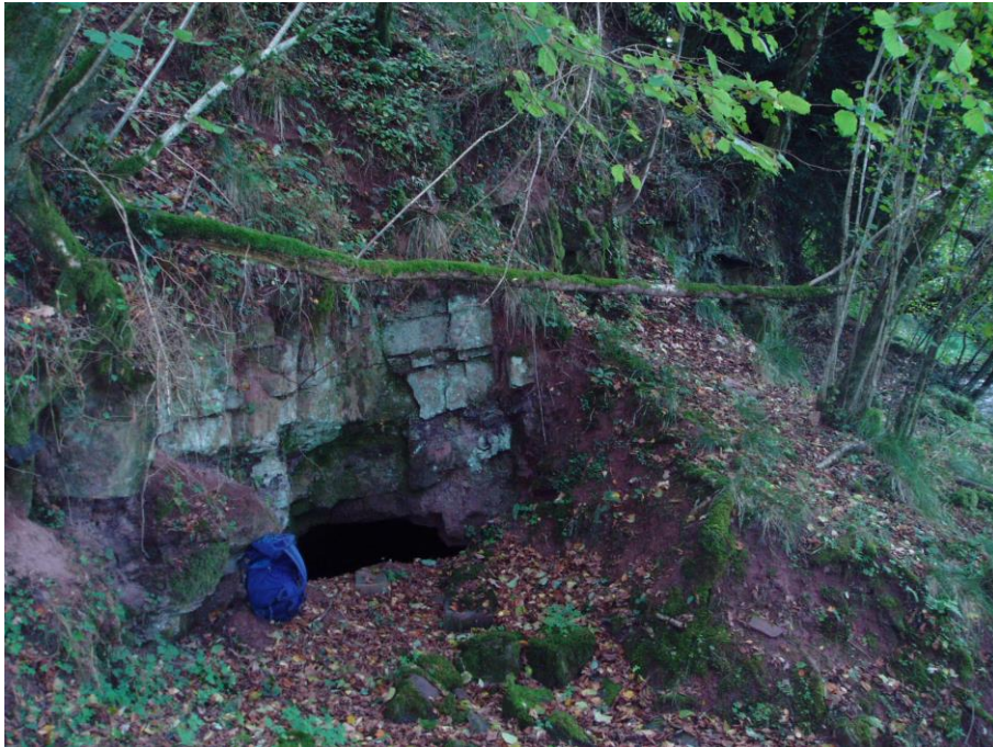
Entrance to adit looking WSW– stream out of photograph to right. Note sandstone bed above entrance
