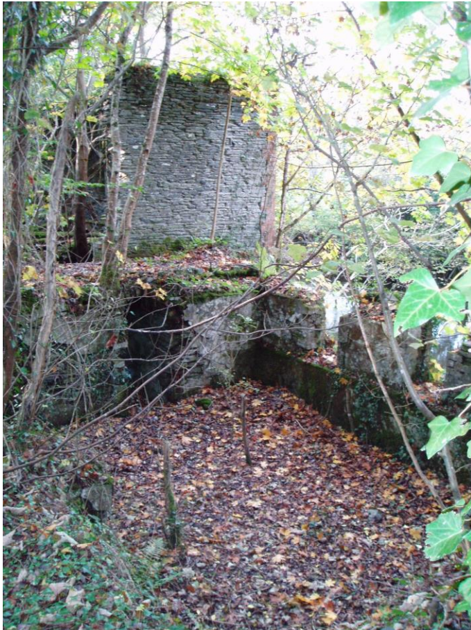
Remains of wellhouse with wall of pump room beyond.
