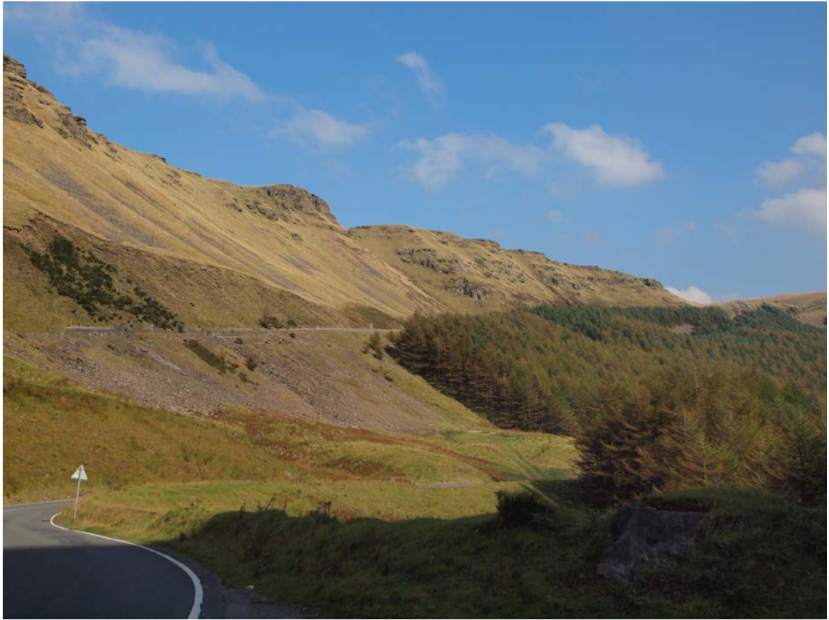
Area of landsliding in middle foreground along lower road
