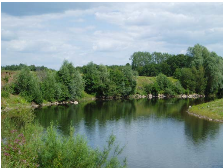
Some large boulders are in place to reduce scour of riverbank
