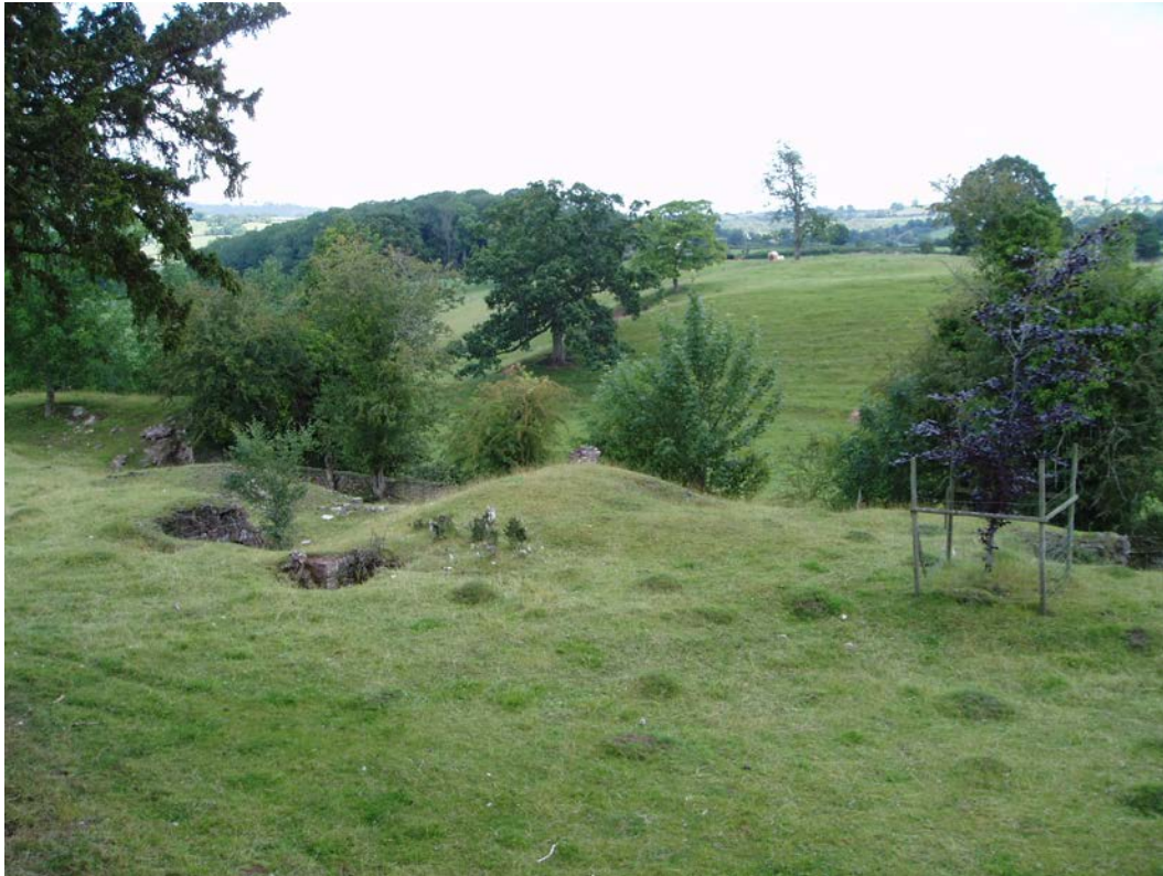
View north-east from churchyard across main channel. On left are the remains of the cellars of Llantilio Court demolished in 1930.
