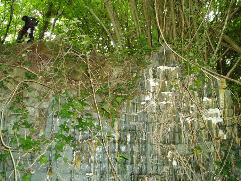
Brickwork on northern wall of blast furnace
