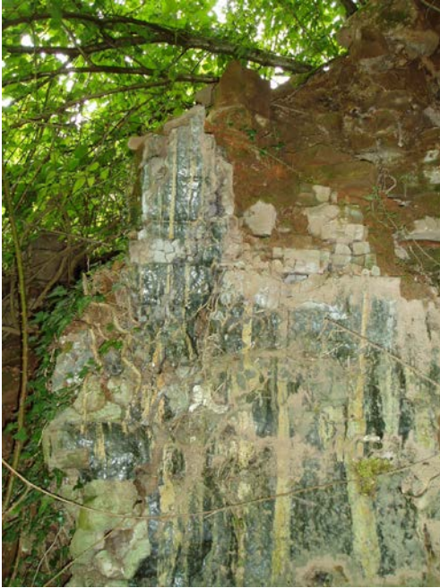
Wall of blast furnace clearly showing iron slag fused to walls. Collapsed charge hole to top right of image
