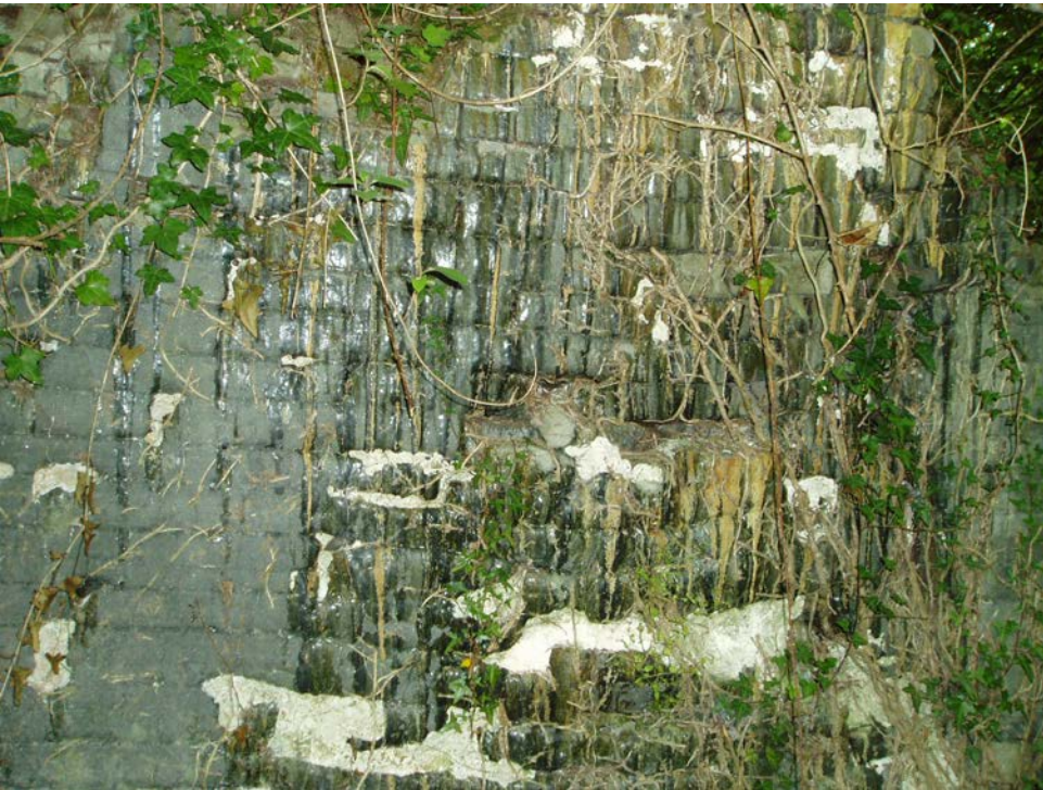
Brickwork in lower half of northern wall of blast furnace
