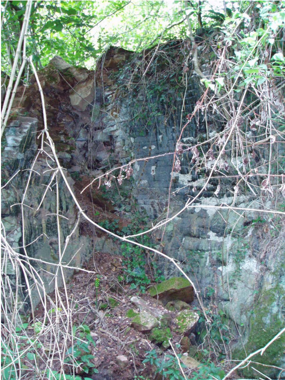
View west showing the overgrown remains of the 17 th Century Coed Ithel blast furnace. The charge hole on the left has collapsed since the 1970's, filling the base with rubble. Note "two cone" internal form of the blast furnace
