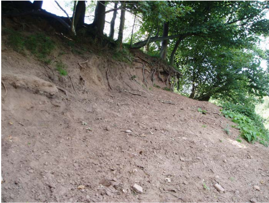
Sandy till dominates on channel margins, but lenses of reworked sand and gravel are visible.
