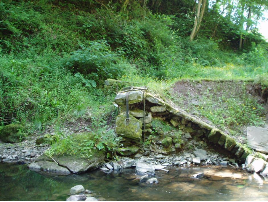
Remains of former Brecon ironworks weir across Afon Honddu
