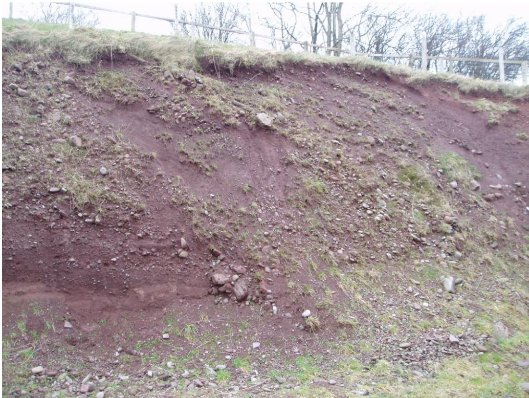
Section shows bedded sands and gravels which have then been disturbed by collapse structures and faulting. The upper part of the section shows evidence of mass movement processes
