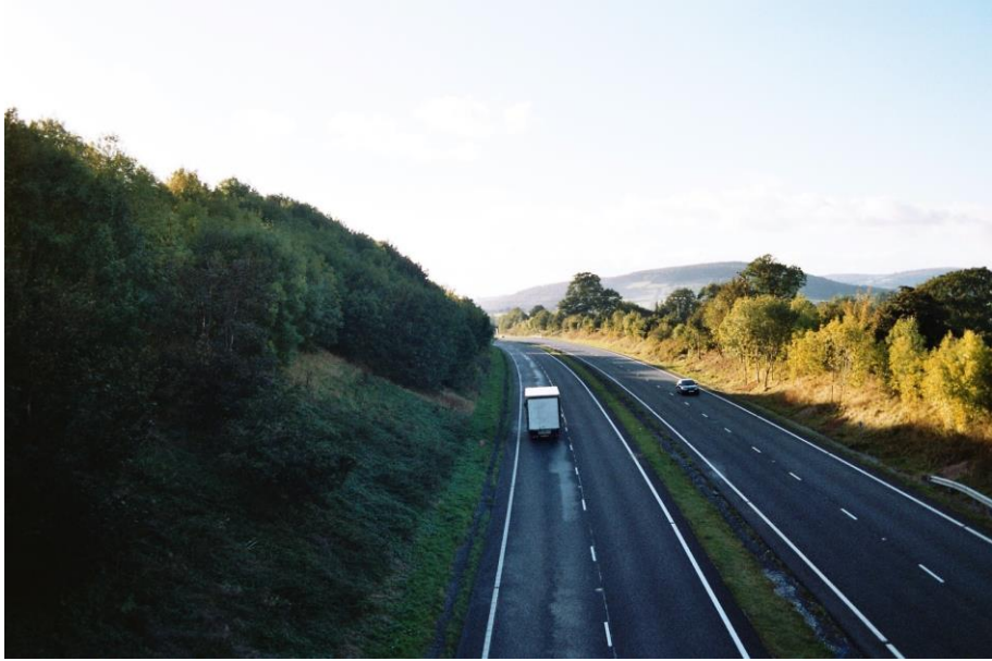
Brecon bypass cutting cuts across morainic ridge feature – view from minor road bridge looking west
