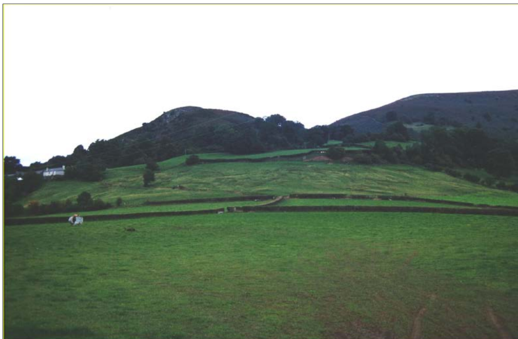
Active shallow translational failures forming distinct features on the slope in the centre of the view. The large mound left of centre on the skyline is the detached translational block part of the main Cwmyoy landslide. Photograph: A. Humpage
