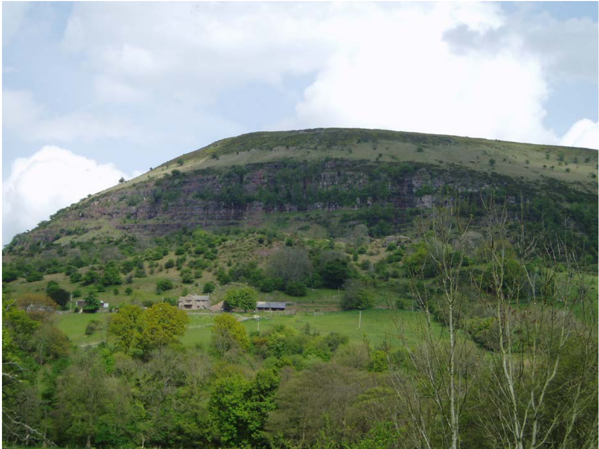
Backscar of the Darren landslide
