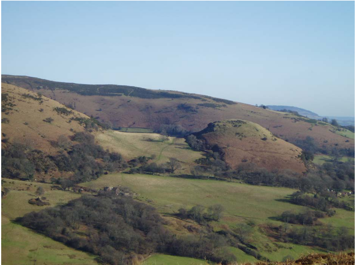
The upper part of the Cwmyoy landslide with large detached translational block – a probable bedding plane failure. View looking south-east.
