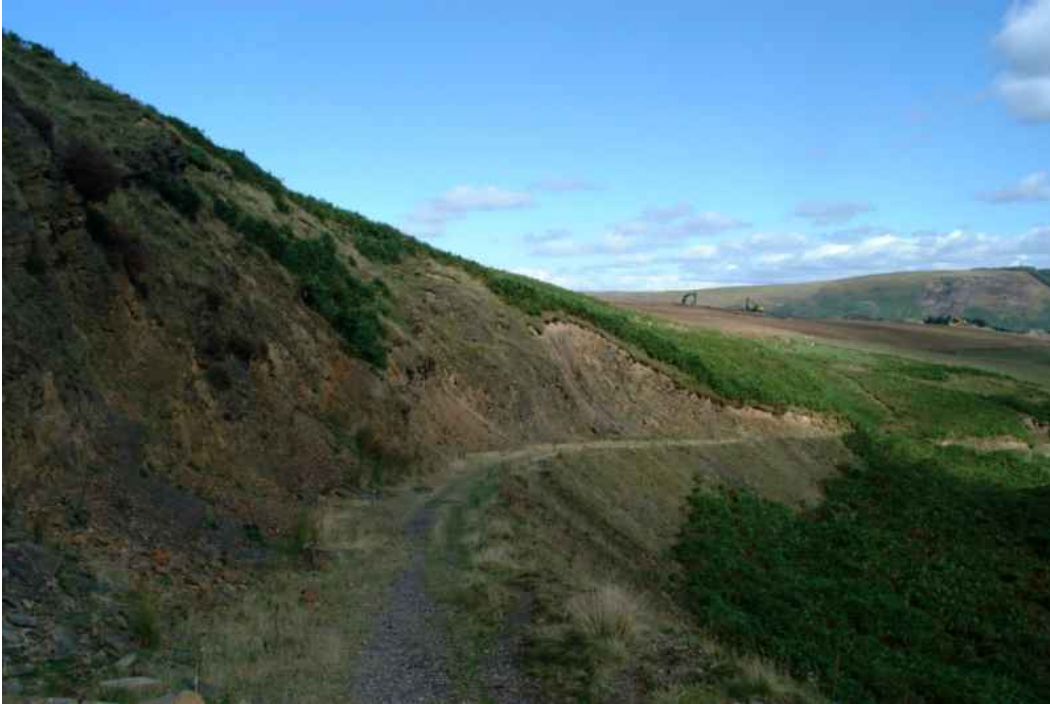
General view of track cutting (Photograph by Andrew Haycock)
