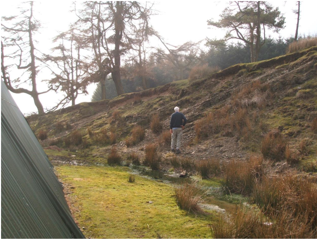
General view of cutting.
