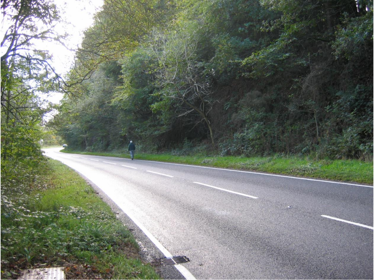
General view of the road section.
