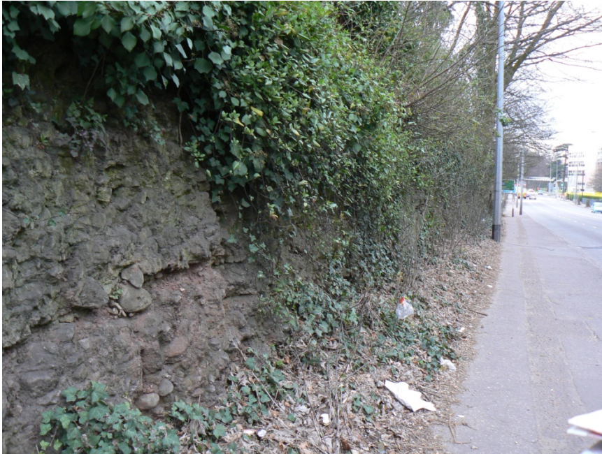
General view of site looking towards the north-east
