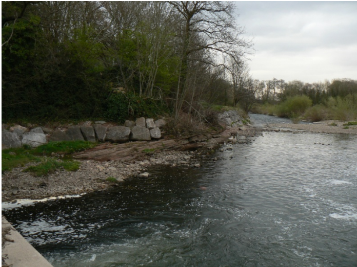
General View of site. North Bank of River Taff looking east
