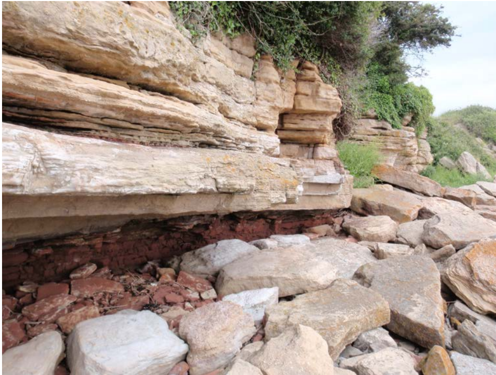
Eastern end of section Sudbrook Point T Sharpe
