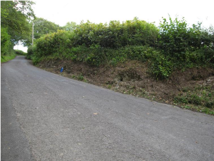
Photograph 1. Cefn Cerig (Fron) road section looking north; cutting on right (east) exposes the contact with the Wormwood Formation (see Photograph 2)
