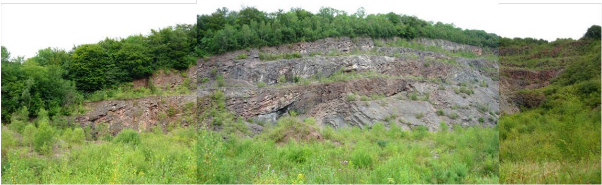
Cefn Garw quarry, panorama of north side, Avon and Pembroke Limestone Groups
