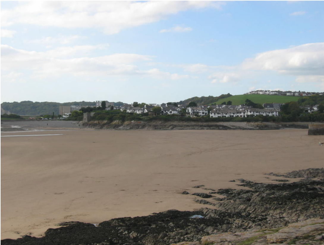
View across Barry harbour showing section in middle distance.
