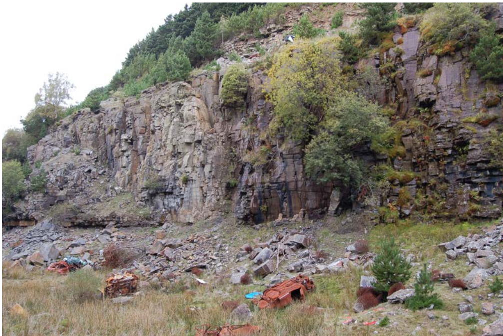
East end of face showing very poor stability of vertical faces, strong master joints, a higher level bench which is not accessible safely and wrecked cars on the floor. Photograph by David Roberts
