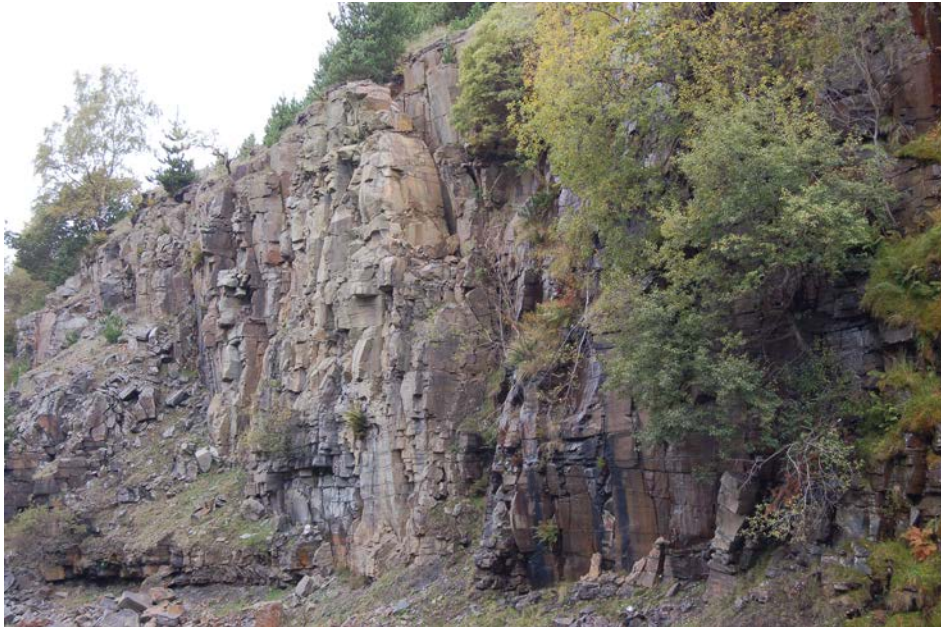
Poor face stability and toppling. Photograph by David Roberts
