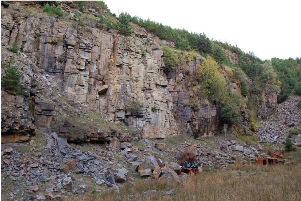
Unstable east end of site showing loose blocks and evidence of recent collapse. Photograph by David Roberts
