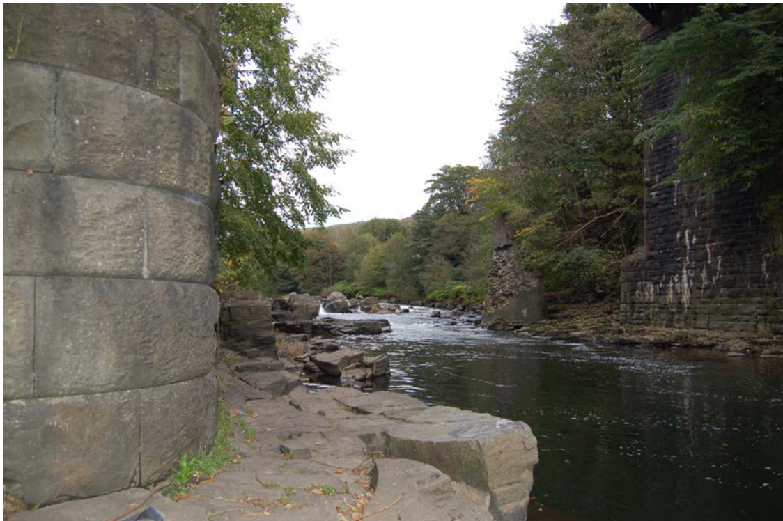
Sandstone base for viaduct pillar, clad with well dressed sandstone: remains of aqueduct pillar are visible on opposite side of river. Photo by David Roberts
