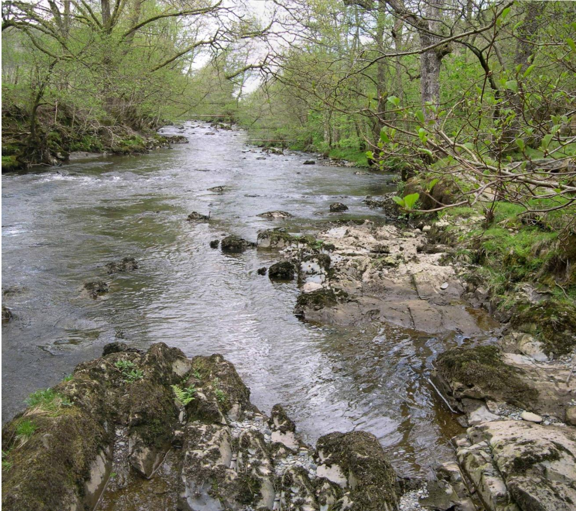
Outcrop in NE bank of River Irfon, viewed towards NW; footbridge in background
