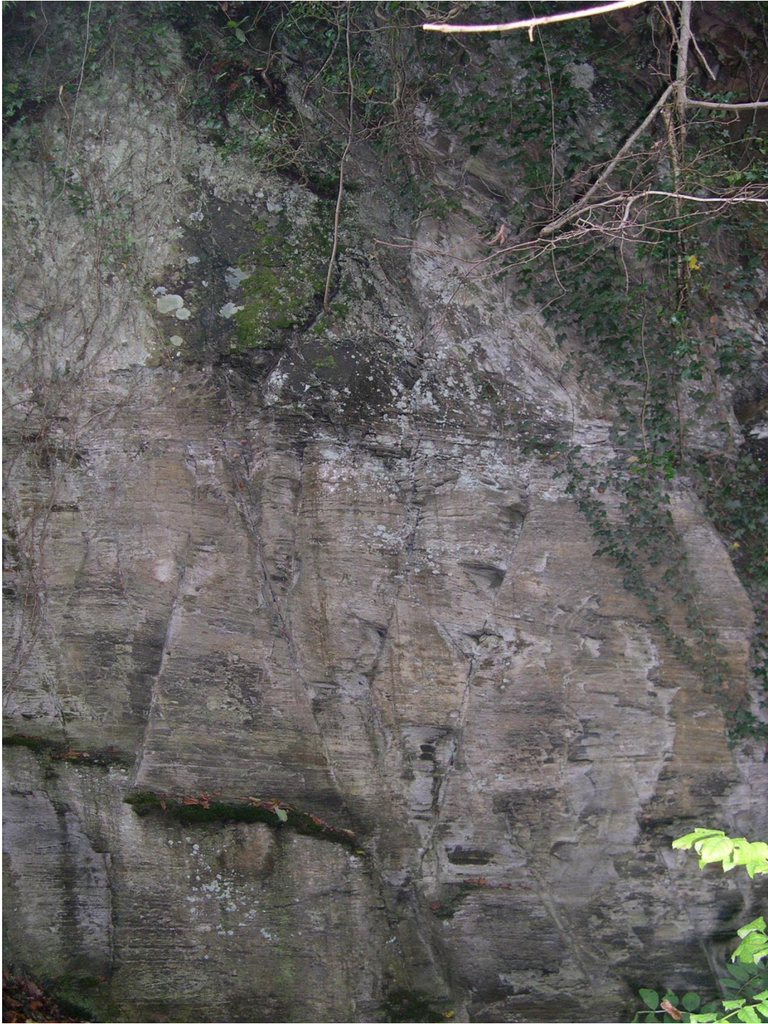
Slump folds, south bank of stream by bridge
